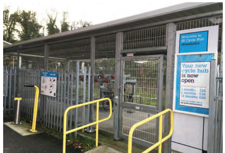
Figure 2 Secure Compound at Greenhithe Station
