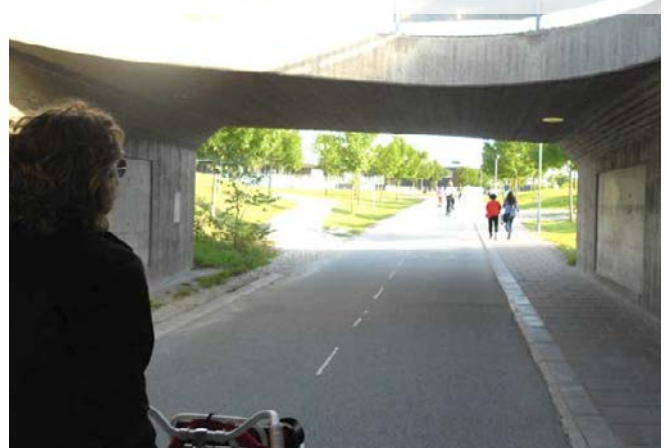
Figure: 10.52 Underbridge (cycle and pedestrian-only) with divided carriageway above to create opening – Lund, Sweden
