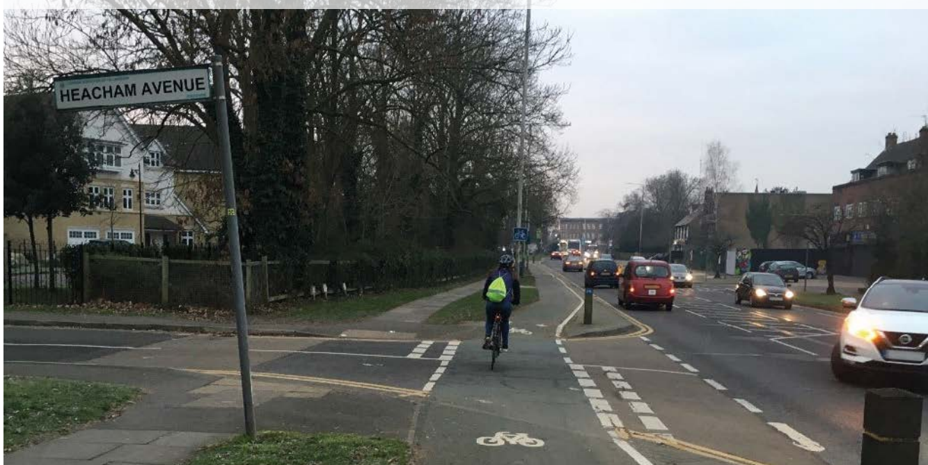
Figure 10.16: Partial set back, marked priority crossing, Hillingdon
