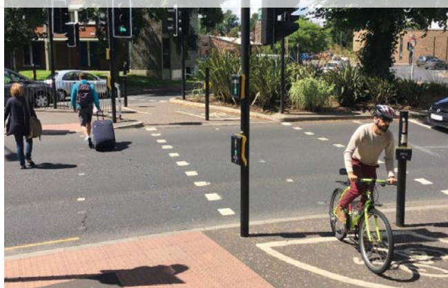
Figure 10.10: Two-stage angled crossing with cycle signals on the central island (Norwich)
