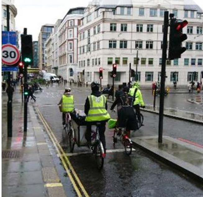
Figure 10.32: Cycle gate, Southwark Bridge, London
