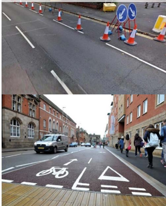
Figure 6.2: Newark Street, Leicester – Trial of traffic lane closure and new two-way cycle track taking the place of the coned-off lane
