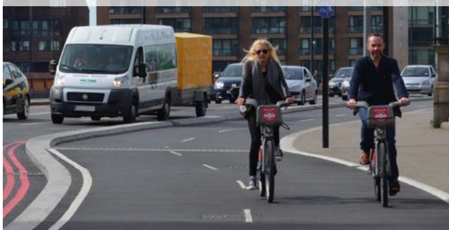
Figure 6.7: Footway level cycle track with raised trapezoidal strip, London
