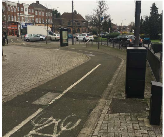
Figure 10.36: Footway-level cycle track around large roundabout, Harrow
