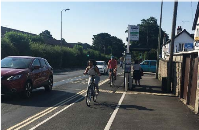
Figure 6.31: Bus stop boarder at quiet suburban bus stop, Oxford
