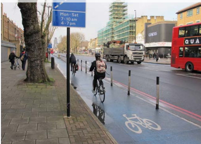
Figure 1.4: Cycle lane incorporating light segregation with flexible wands
