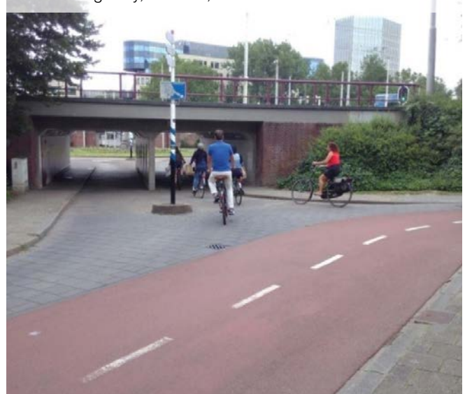
Figure 10.48: Cycle and pedestrian route grade separated from carriageway, Arnhem, Netherlands
