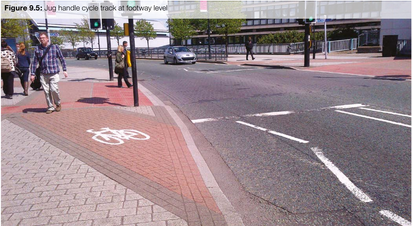
Figure 9.6: Stepped cycle track diverges from carriageway, Gateshead
